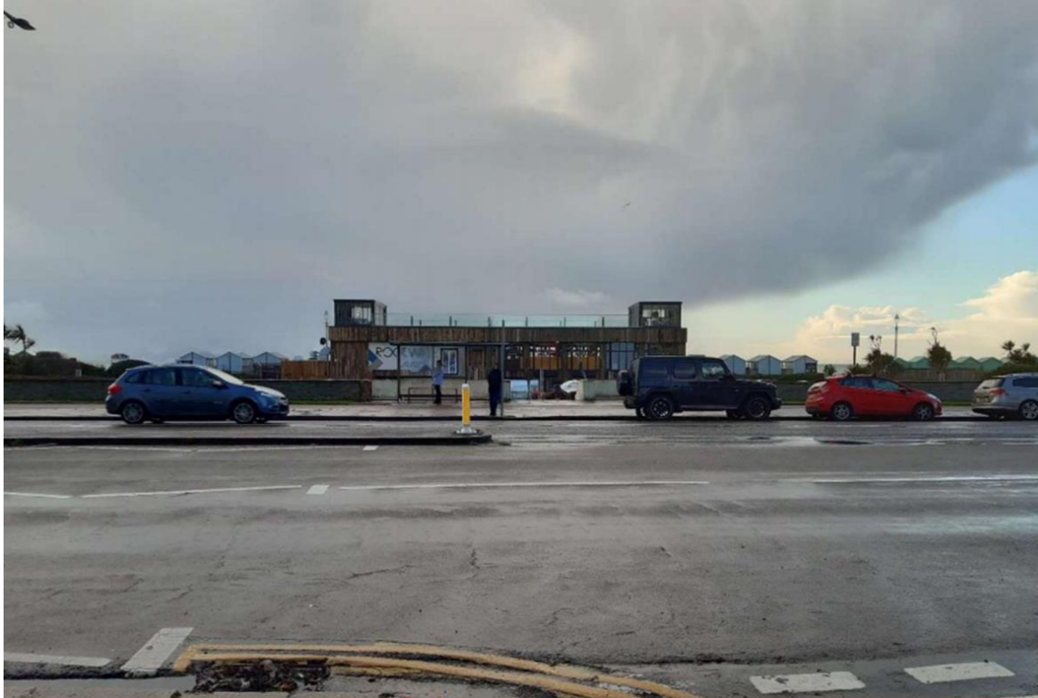
Photo taken from the north side of Kingsway (A259) on 06.12.2020
